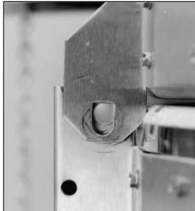
Notice the  $\frac{1}{16}$ " gap in the lid and the position of the slotted hole.
