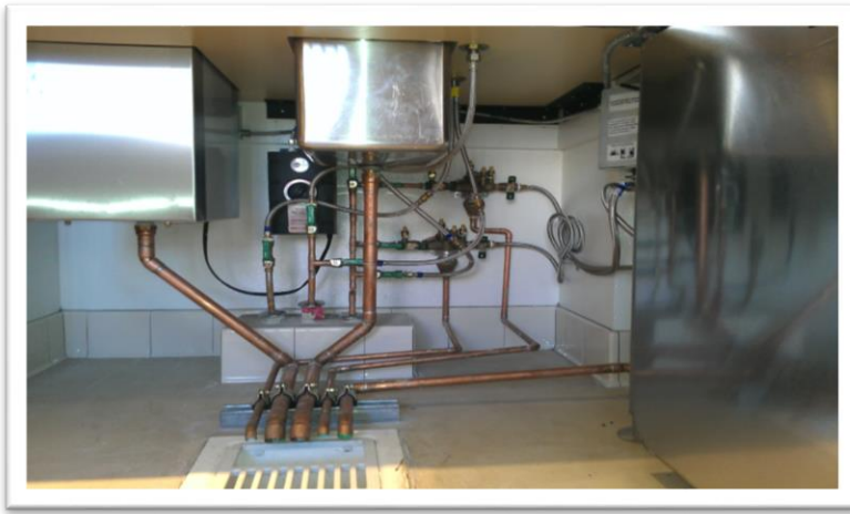
Fig. 8 Indirect Drainage of Waste to a Floor sink
